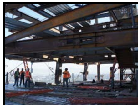
Structural Steel Erection
