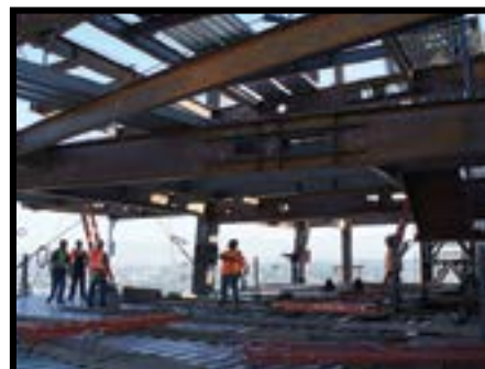
Structural Steel Erection
